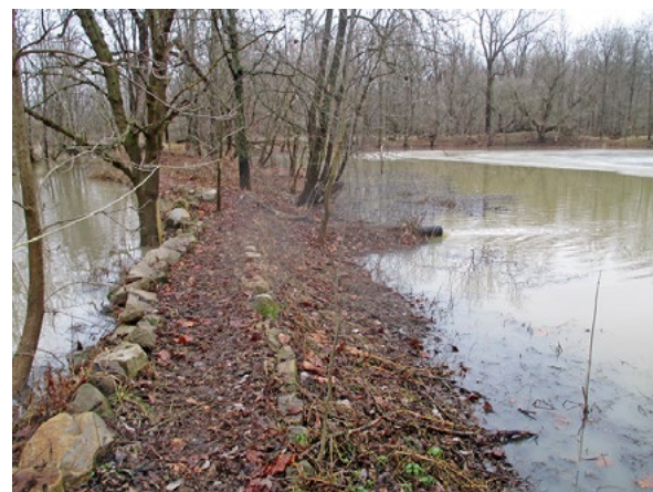
The view from David's Landbridge: As Cranberry Run (left) flowed merrily with December rain, the quarry (right) finally filled after two dry seasons.
